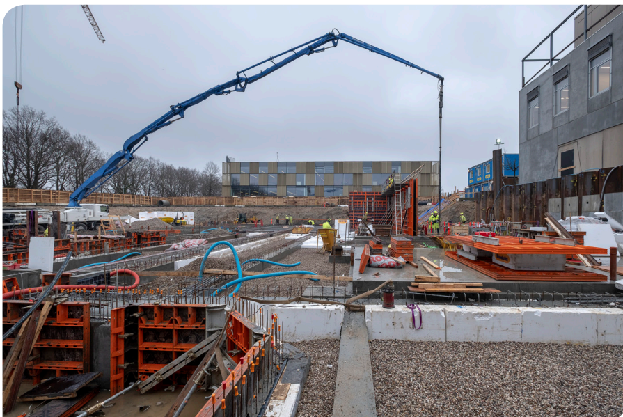
Below: The new DTU Headquarters, built partly with FUTURECEM™. Source: Torben Eskerod.
