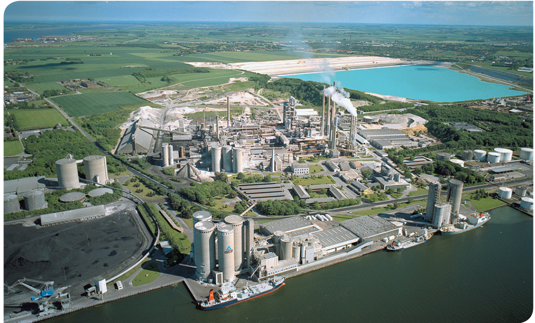
Right: A view of part of the Aalborg Portland cement plant in Aalborg, Denmark, where the Cemistir Research and Quality Centre is based.
