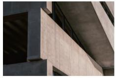
FUTURECEM® has been used in RMC for total 4,880 m² Bjarke Ingels Group HQ office which is set to achieve DGNB Gold. Through use of Uni-Green – a new type of concrete by Unicon based on FUTURECEM® technology that has a CO2 reduction of approx. 25%, resulting in a CO2 footprint of 11.3kg CO2 eq/m²/year.
